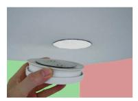
Now simply place the smoke alarm on the ceiling element.
